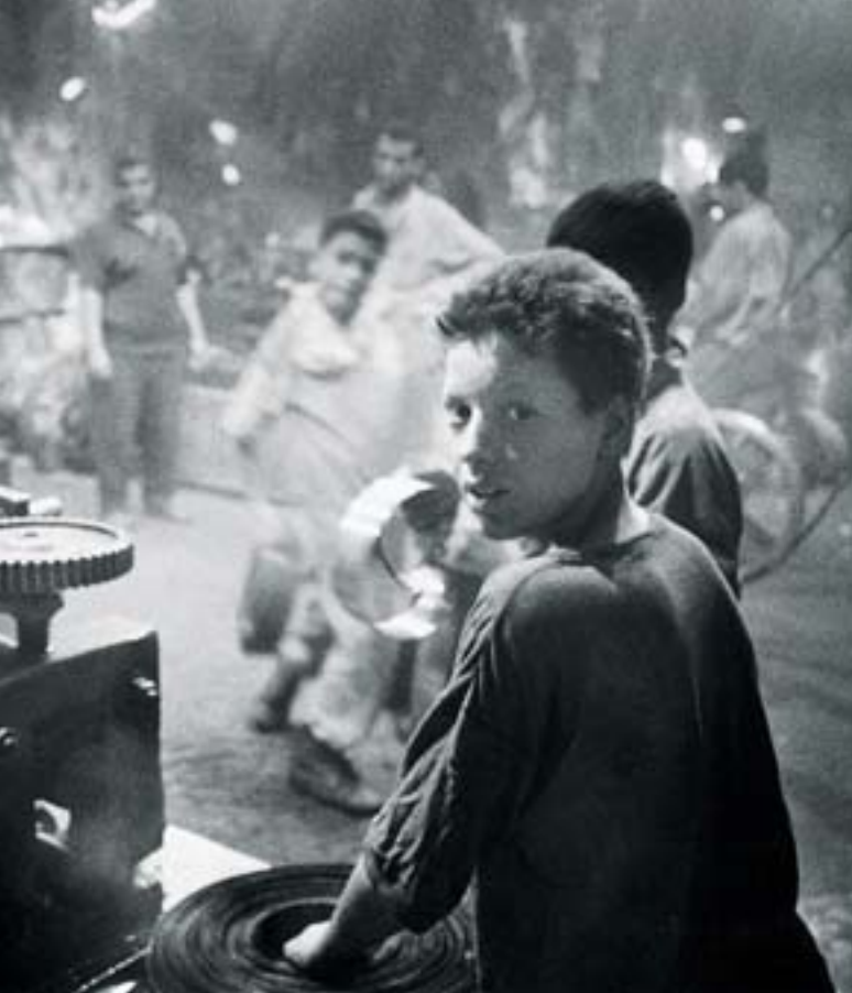
STEEL PRODUCTION PLANT, Cairo, Egypt
