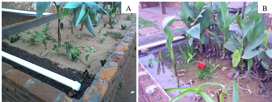
Figure 2 Constructed wetland (school). A: before start up. B: after 5 months of operation, problems with clogging and overflow.
