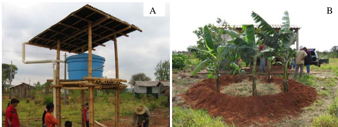
Figure 1 A: rain water harvesting system (bamboo structure) for one household. B: banana tree circle (permaculture) at a communal laundry area.
