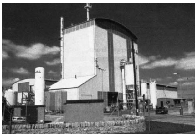
Figure 8.1 Eggborough gasification plant.
