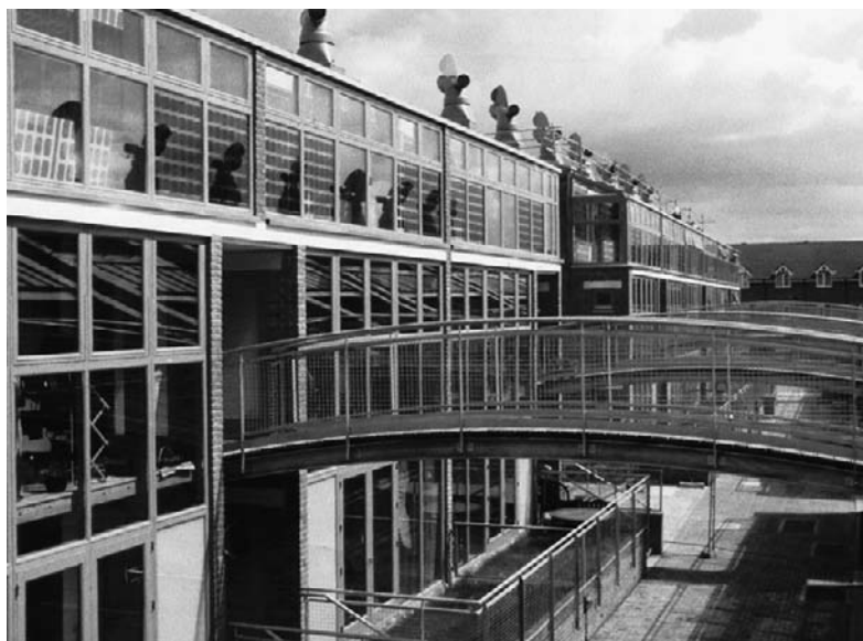
Figure 15.16 South elevation with PVs integrated into the glazing.
