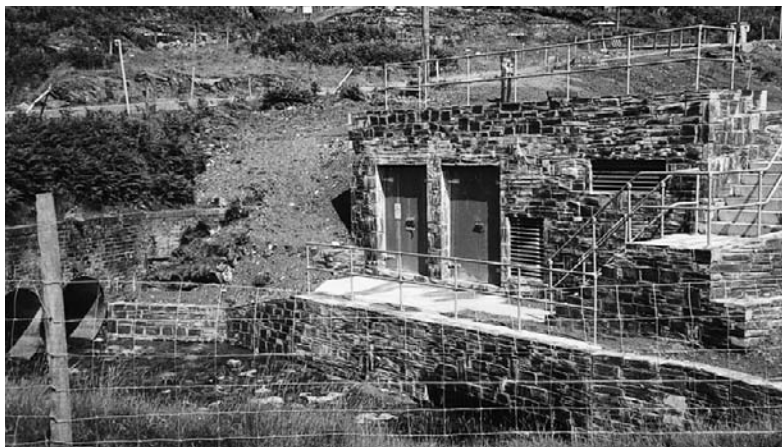
Figure 10.1 Ffestiniog small-hydro plant, Tanygrisiau, north Wales.
