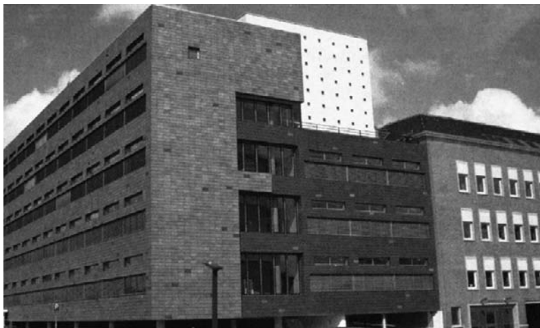
Figure 15.6 Enschede Tax Office extension, the Netherlands.
