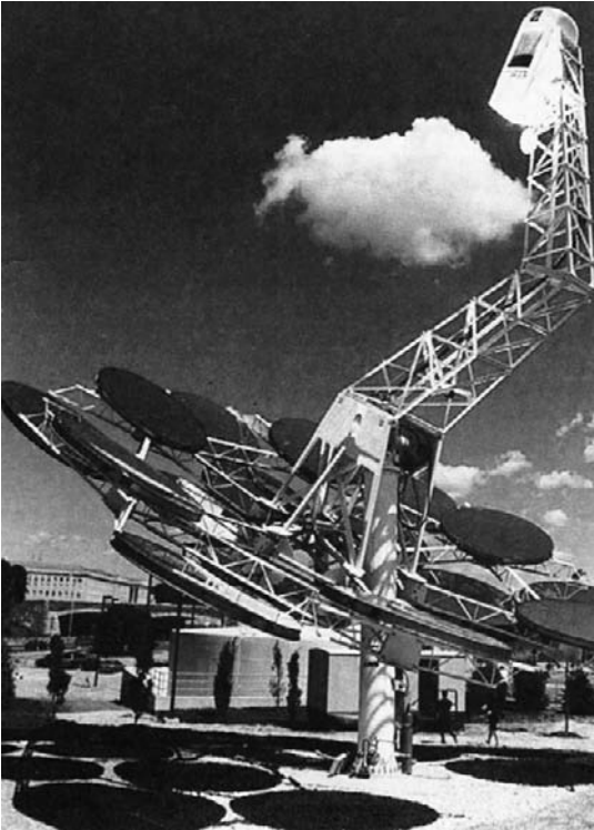
Figure 2.17 Parabolic Sundish with Stirling engine the 'Powertower' in the USA. (Courtesy Renewable Energy World .)
