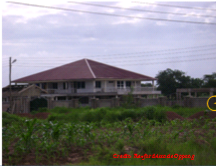
Vice-Chancellor's Lodge under construction as at June, 2008 on the Tamale Campus of the University of Development Studies in Ghana roofed with anodised aluminium sheets .
