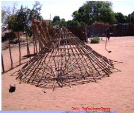
Locally constructed roof structure of wood saplings in Mukuni Village
