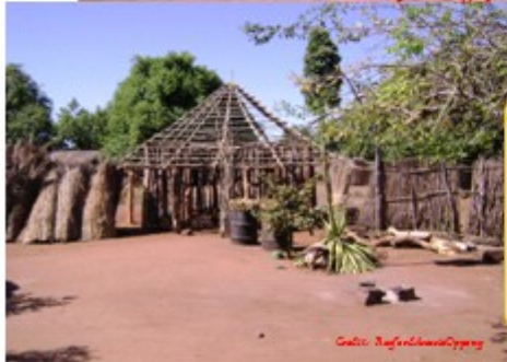
Roof structure to receive thatch roof covering in Mukuni Village compound
