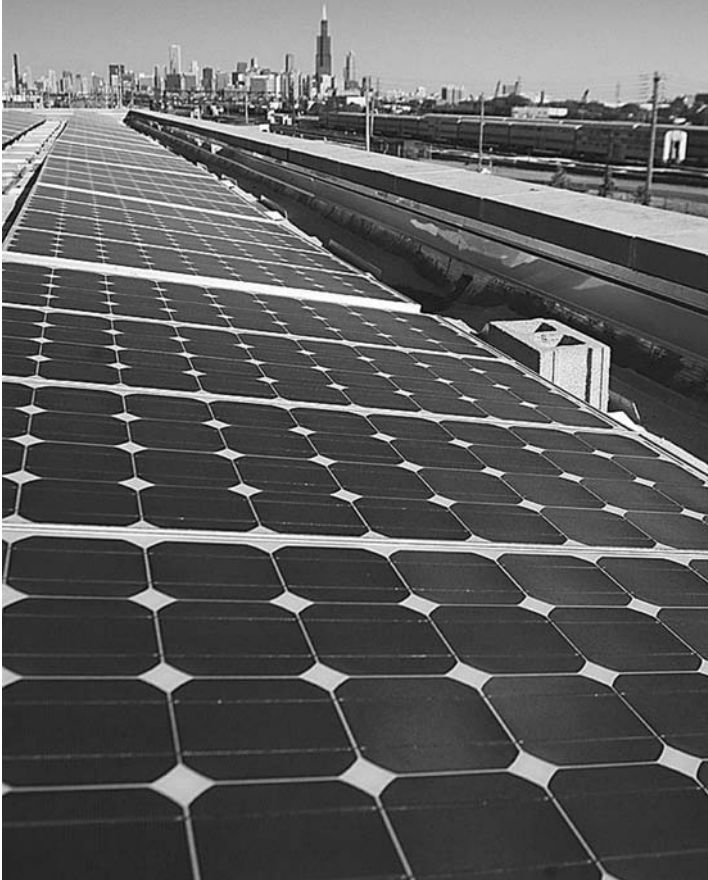
Figure 15.1. Farr Associates' Chicago Center for Green Technology has a rooftop photovoltaic system. © Farr Associates Architecture | Planning | Preservation, Chicago, Illinois. Photo by Chris Kelly.
